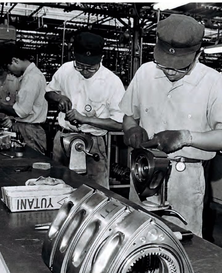
The manufacturing of the rotary engines requires a high amount of precision.
